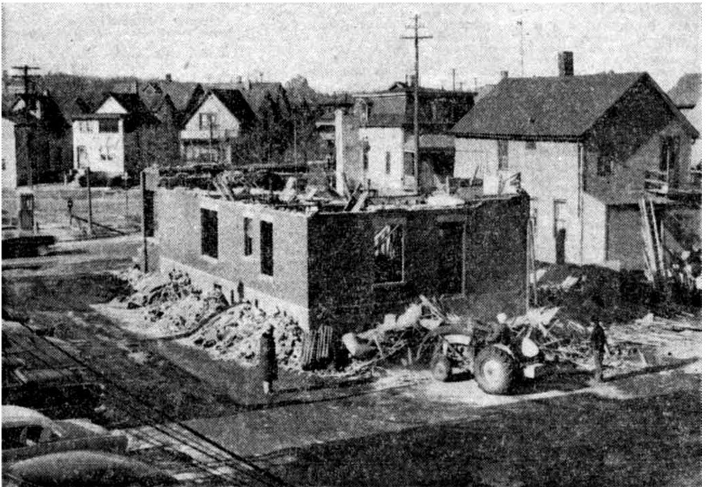
"Demolition of buildings bought by the city under the Brittingham redevelopment program became strikingly evident when this brick apartment house on West Washington Avenue started to disintegrate under the wreckers' hammers. Here a crewman of the Allen Wrecking Company operates a power shovel to pick up debris while his helper and a bystander look on."
