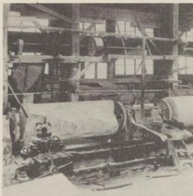
Left, Column turning lathe, Woodbury Granite Company. Right, Fluting machine. (Both photos: First Church of Christ, Scientist, Boston. )
